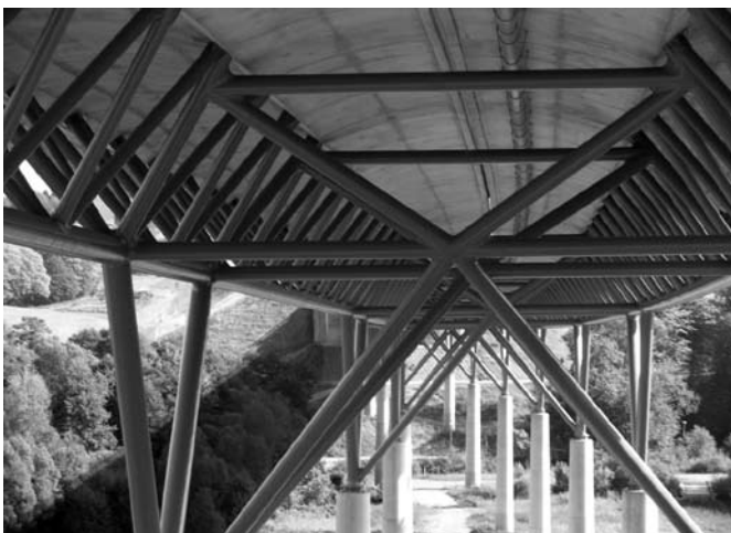
Pipe geometry of the road bridge at Sankt Kilian
