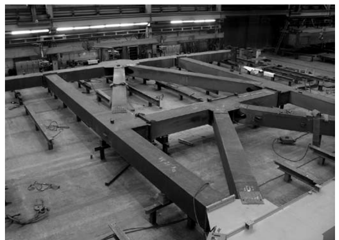
Boiler frame structure for a power station block
