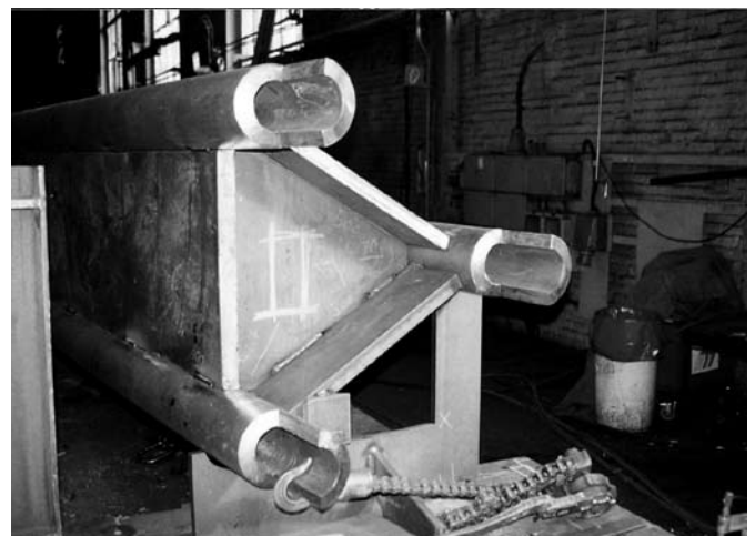
Truss weld seam preparation
