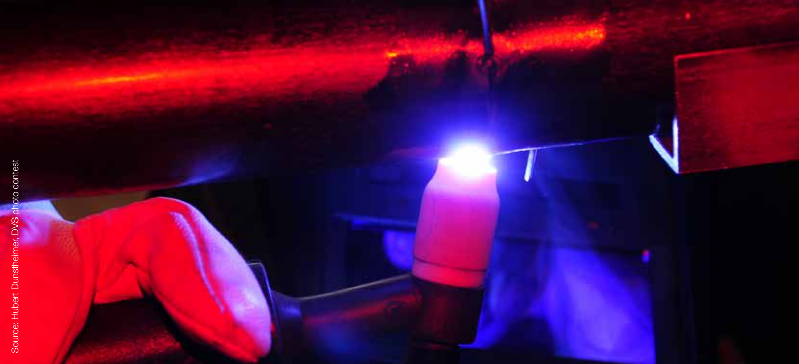
Pipe coupling with TIG welding.
